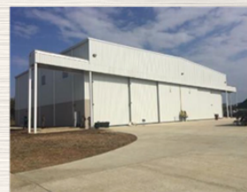
CN/SC Hangar, Nicanor, Panama
