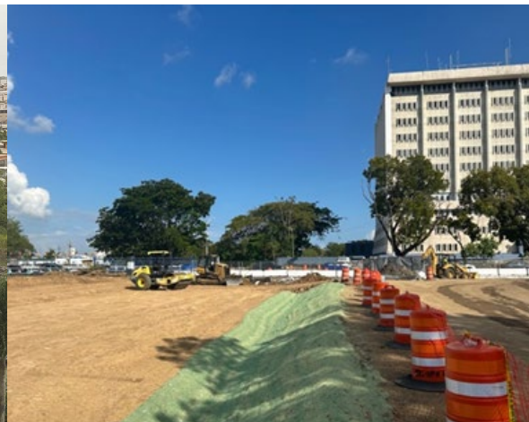
Rio Puerto Nuevo CNT-2 Roosevelt Bridge Replacement
