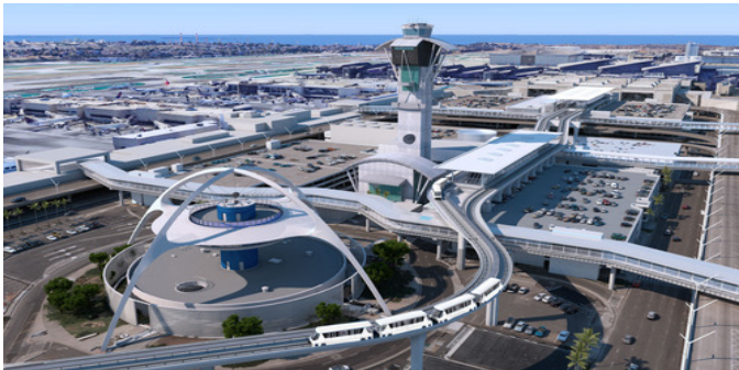
LAX Automated People Mover // Los Angeles, California
