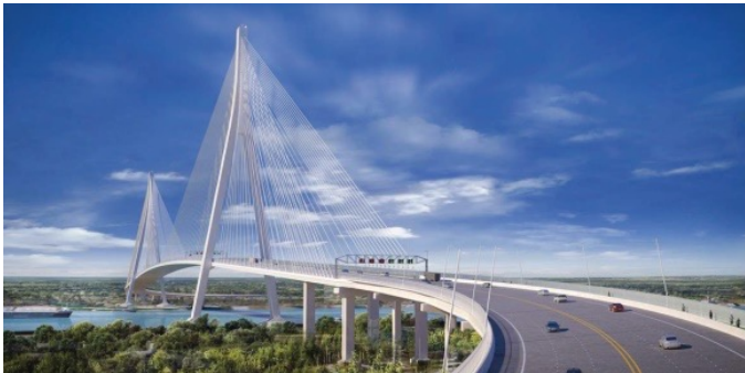
WDBA Gordie Howe International Bridge // Detroit, Michigan and Windsor, Ontario
