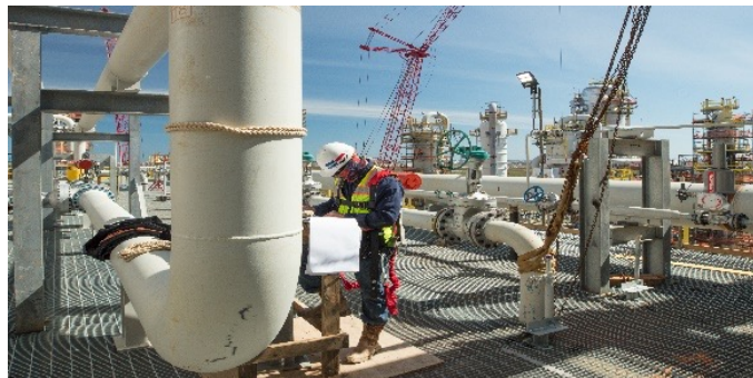
MEGlobal Monoethylene Glycol Project // Freeport, Texas
