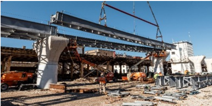
CTA Red and Purple Line Modernization // Chicago, Illinois
