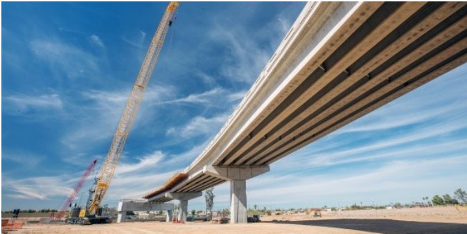
ADOT Loop 202 South Mountain Freeway // Phoenix, Arizona
