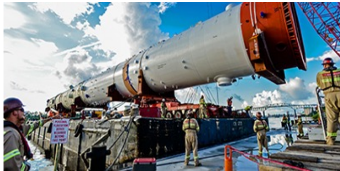
Sasol Ethane Cracker and Derivatives Project // Westlake, Louisiana
