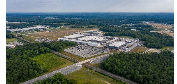
Novo Nordisk API Manufacturing Facility // Clayton, North Carolina
