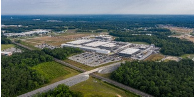
Novo Nordisk API Facility // Clayton, North Carolina
