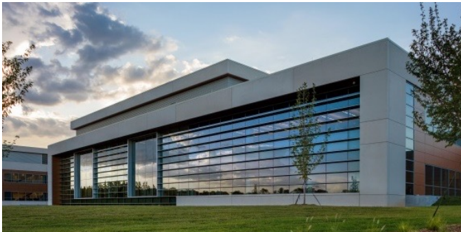
Takeda Biologics Facility // Covington, Georgia
