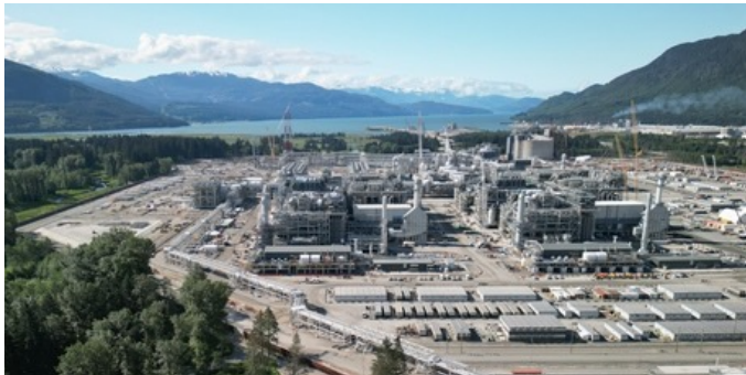
LNG Canada Export Facility // Kitimat, British Columbia
