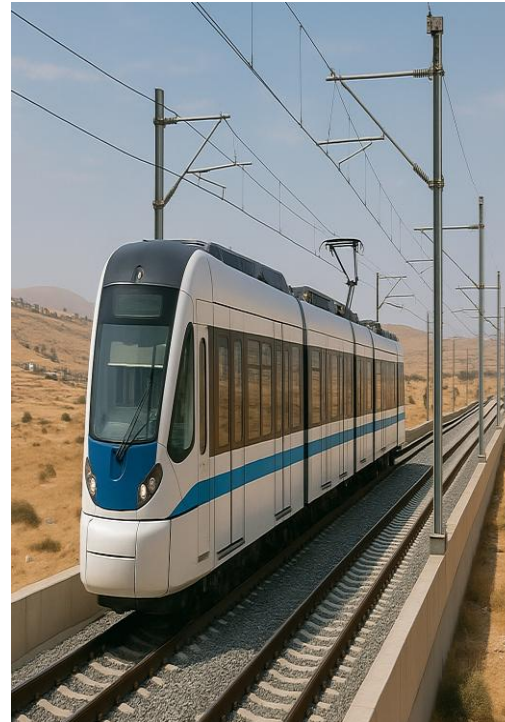
LRT Light Rail Transit (Amman– Zarqa)
