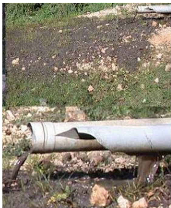
Zibar Wastewater Project
