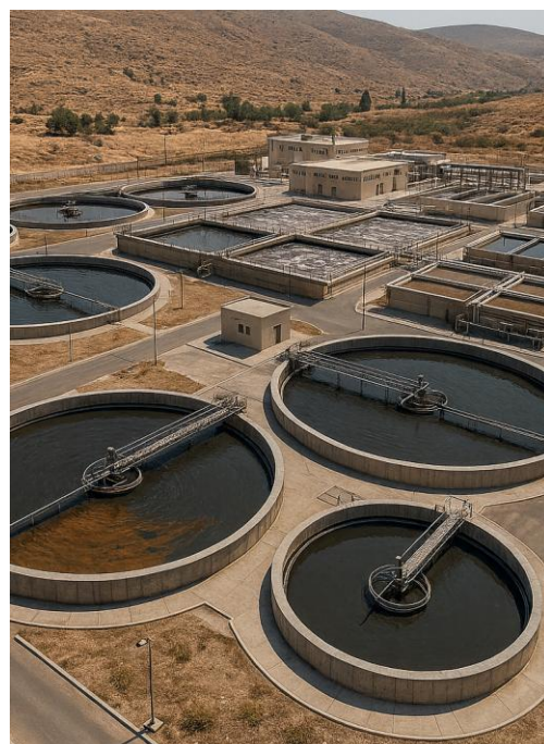
Al-Shallalah Wastewater Treatment Plant
