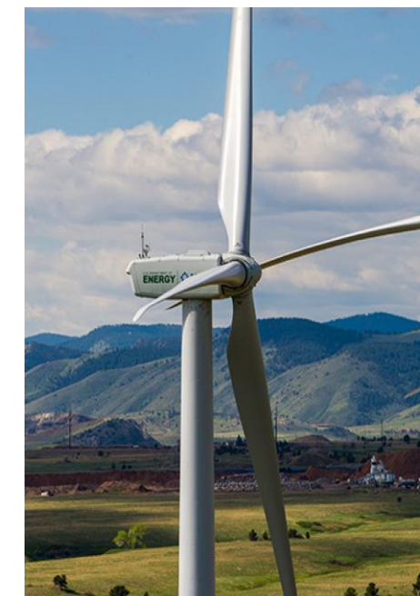
Wind power generation
